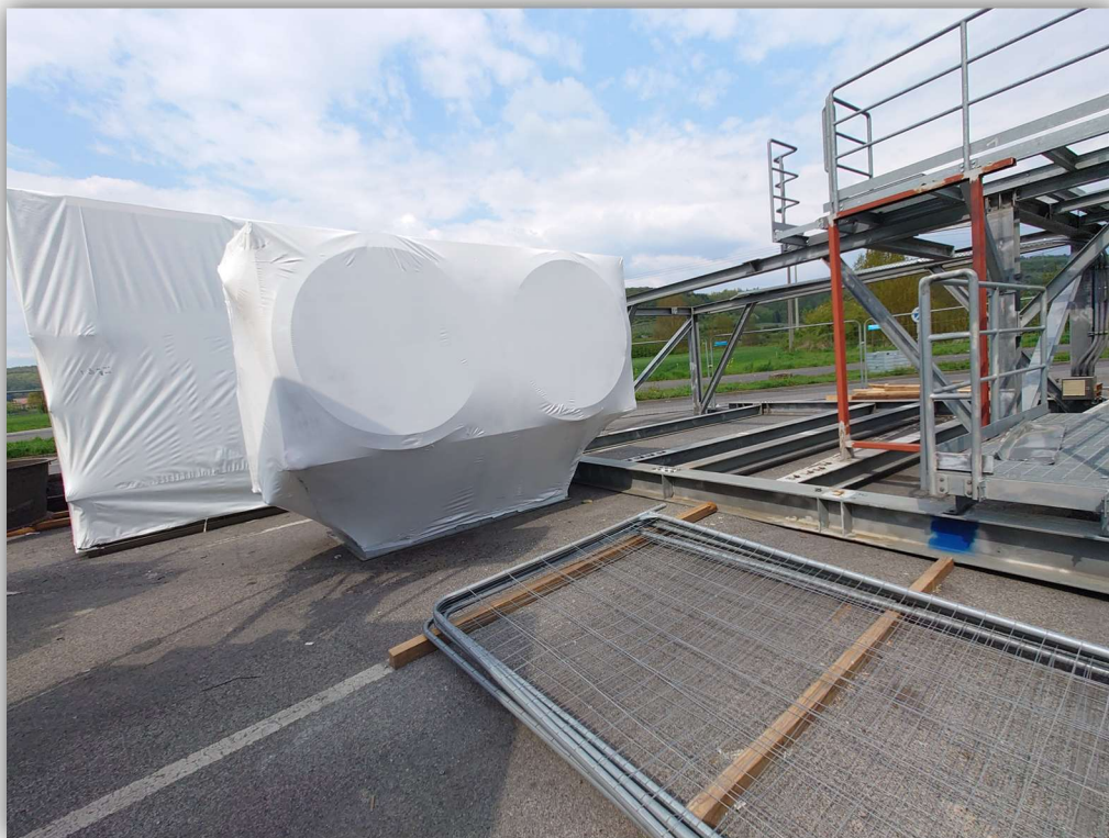
Gas Turbine air system – ready for transport after dismantling
