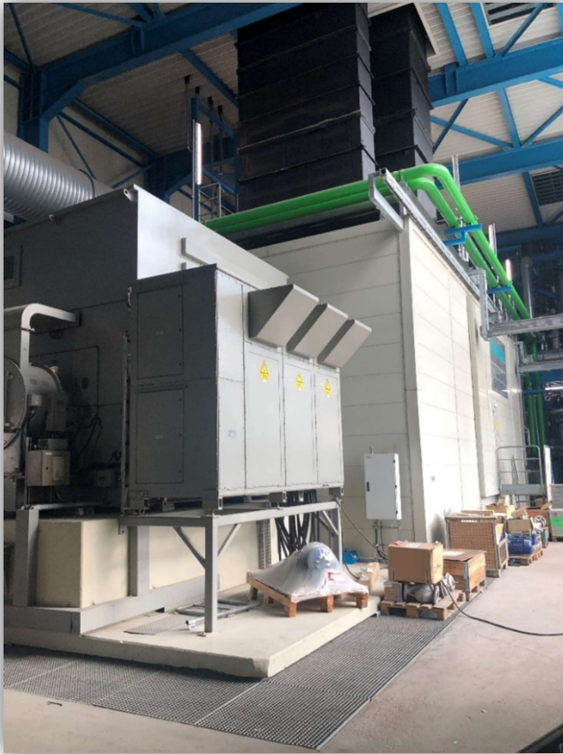
Gas Unit – Side view of the generator and gas-turbine canopy in the back
