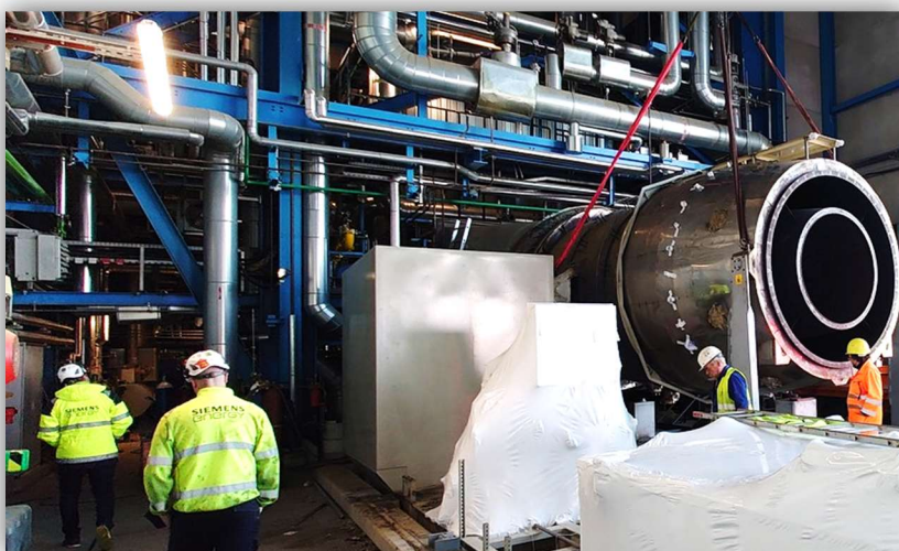
Gas turbine – SIEMENS experts conducting dismantling works
