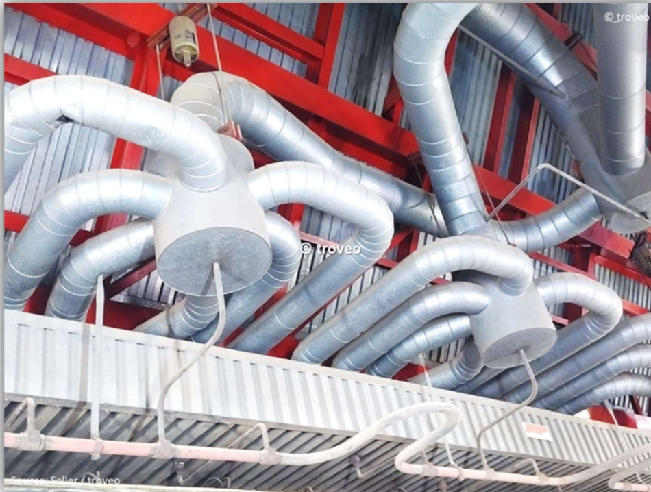
steam boiler – base piping system
